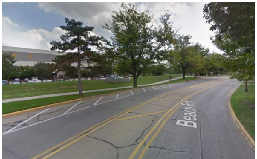
Figure 8: Beach Road has a significant amount of under-utilized pavement space, including striped shoulders and striped medians.
