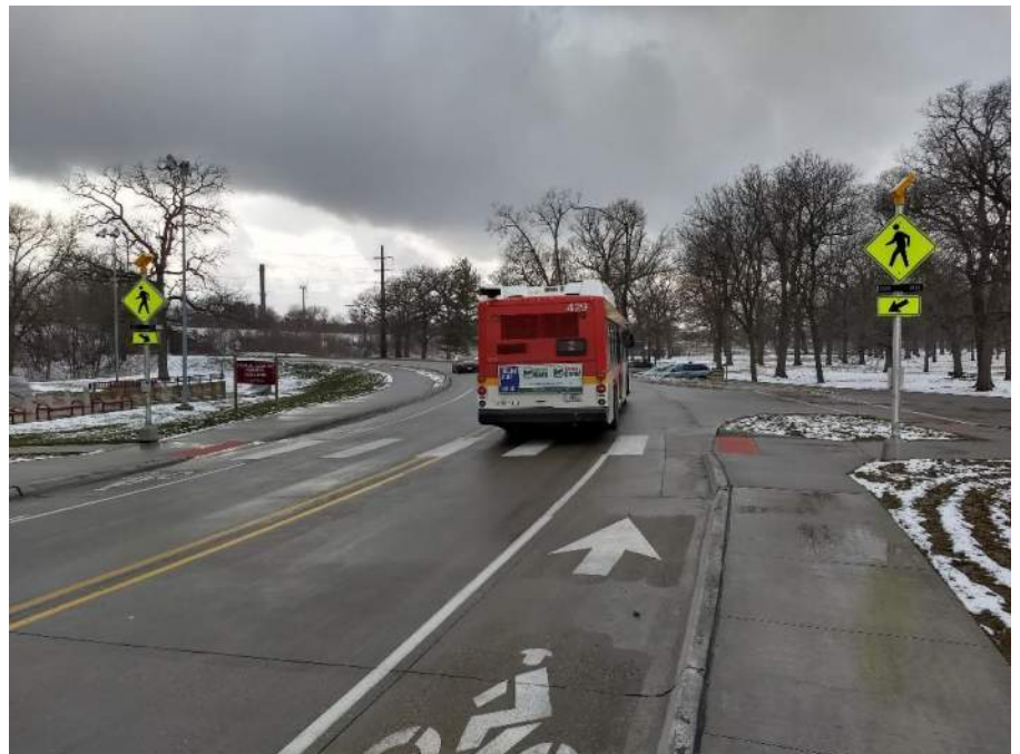
Figure 6: Osborn Drive could have a dedicated bike lane while still accommodating buses, similar to the roadway configurations on 6 th Street in Ames shown above.
