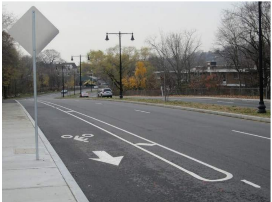
Figure 4: A buffered bicycle lane provides additional space between motor vehicles and bicyclists.
