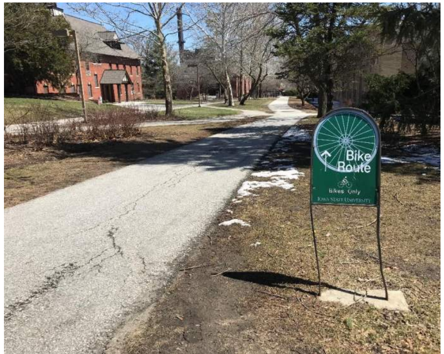
Figure 1: The bike route signs on campus are aging, and the only bike-only path on campus does not have any pavement markings to indicate that it is intended for bicycle use only.
